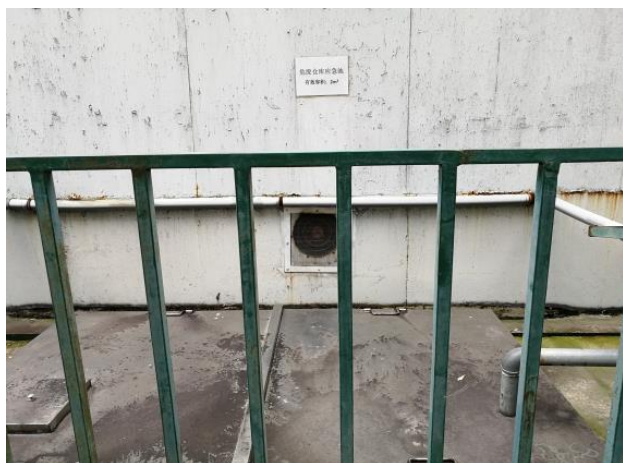
危废仓库应急池 (2m 3 )
